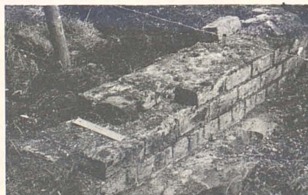
Remnant of one of the brick walls of the drying Kilns.
