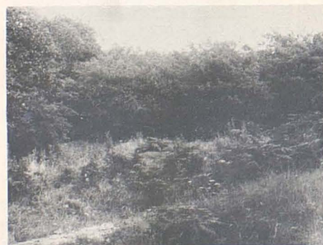
Hodgson's Briquette Factory. The site before excavation.
